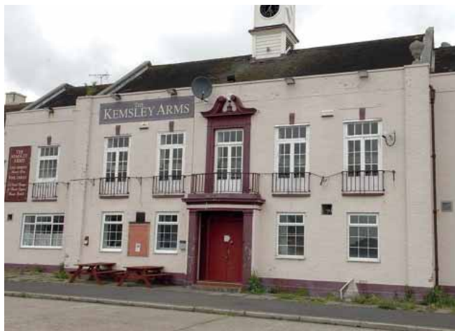
The Kemsley Arms Public House (prior to its closure and deterioration – see baseline HAR register of Appendix II).
