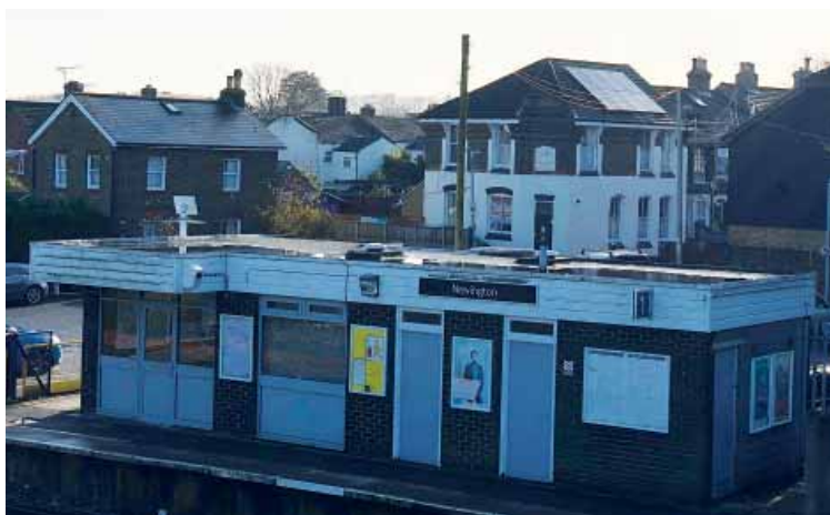
The modern replacement station and adjacent Victorian housing at Newington.
